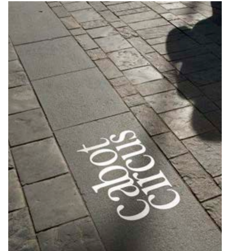
METAL AND STONE INLAYS OFFER POTENTIAL FOR ATTRACTIVE SIGNAGE IN STEPS AND PAVING
