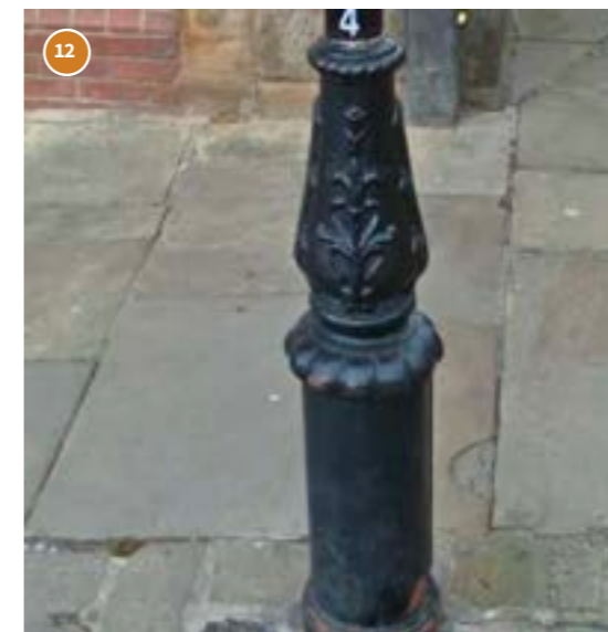
12 TRADITIONAL DETAILING TO BASE OF SOME COLUMNS
