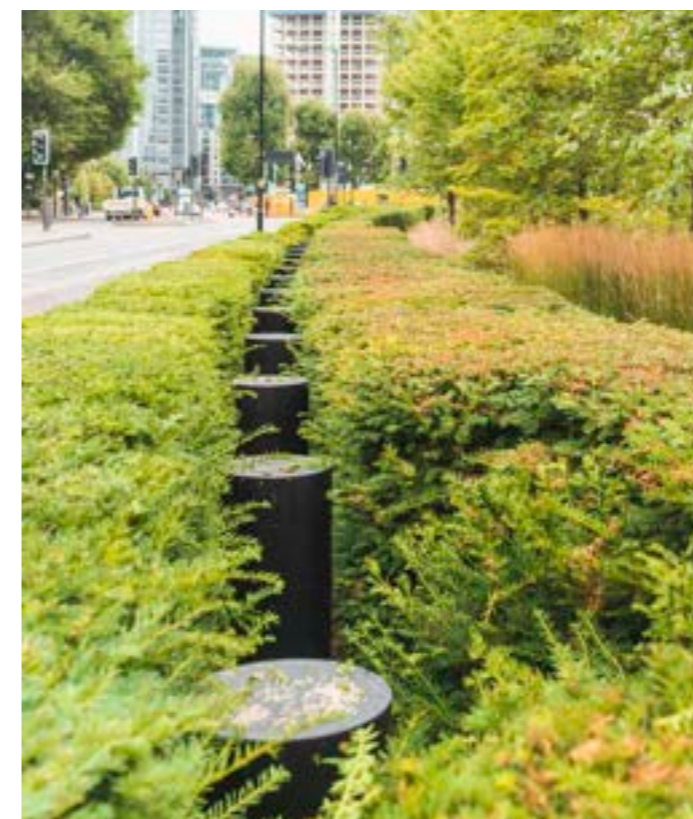
BOLLARDS CONCEALED IN HEDGING
