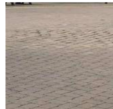
HERRINGBONE CONCRETE PAVERS AT RYKNELD SQUARE
