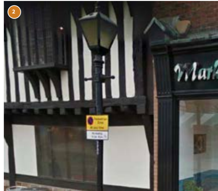
2 HERITAGE STYLED LIGHTING COLUMNS
